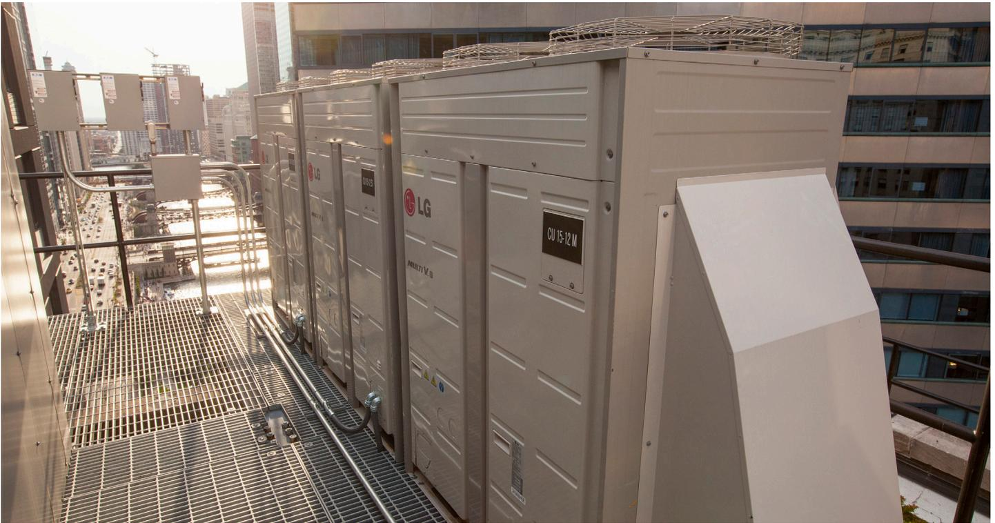
**WITH VRF TECHNOLOGY, THE BUILDING CAN TAKE ADVANTAGE OF RECOVERED WASTE HEAT – THE CAPTURING OF HEAT ENERGY NORMALLY DISCHARGED TO THE ATMOSPHERE BY ZONES IN COOLING MODE AND MOVING THAT ENERGY TO THE ZONES THAT NEED HEAT – SO ONE GUEST CAN HAVE HEATING AND ANOTHER COOLING SIMULTANEOUSLY.**
